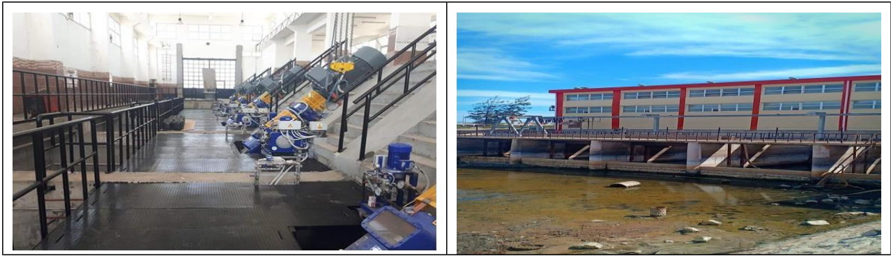
Figure 1: New Faraskour drainage Pumping Station.
